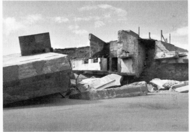
Remains of the eroded Godwin Battery.
